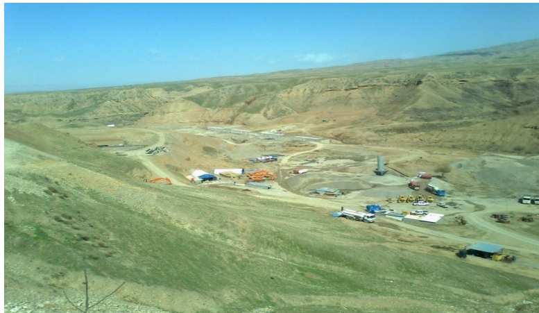
Figure 15. Reservoir area during preconstruction phase (MAWR, 2010).
