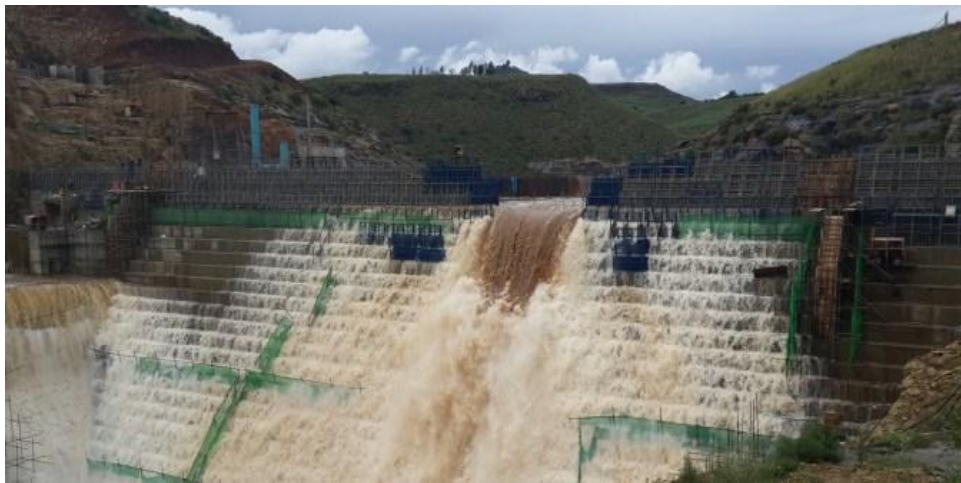
Figure 2. The Metolong Dam is overtopped due to high inflow sedimentation in March 2014. Lethoso- South Africa. ( http://www.engineeringnews.co.za/article/lesothos-metolong-dam-close-to-completion-2014-05-05 ).
